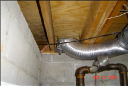
Disconnected duct
